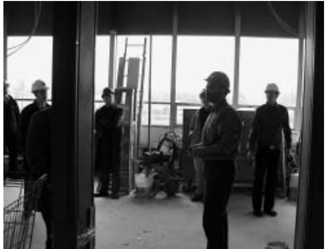
Construction tour of the Carter Center for Music Education.
